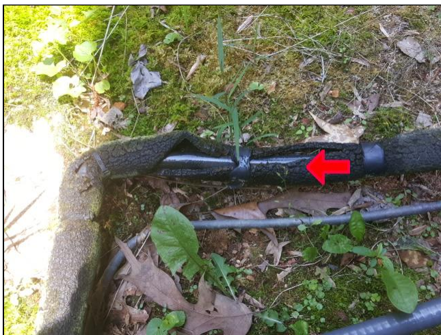
8.7 Item 1(Picture) Tube Deterioration
