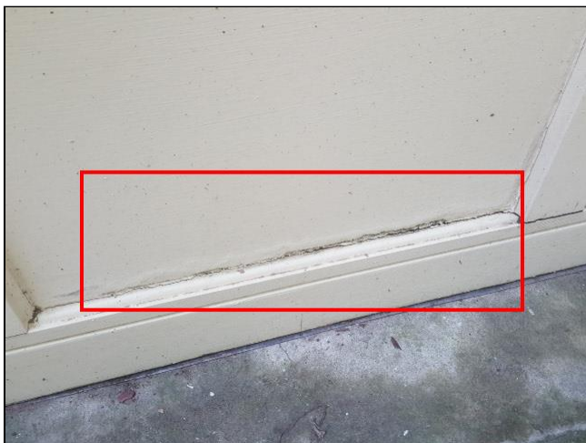
3.3 Item 1(Picture) Moisture Damage
