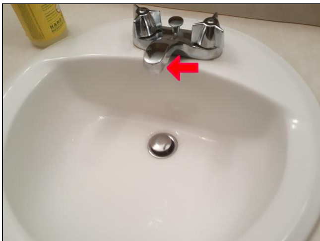
6.1 Item 1(Picture) Valve Leak
